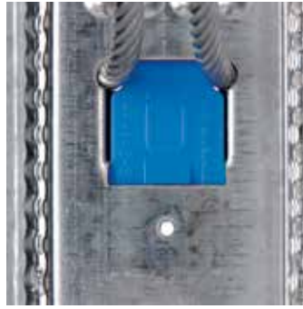
Figure 12: ISI identification with blue clip
